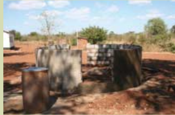
Walls for the new kitchen
