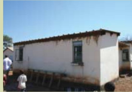
Refurbishment of headteacher's house
